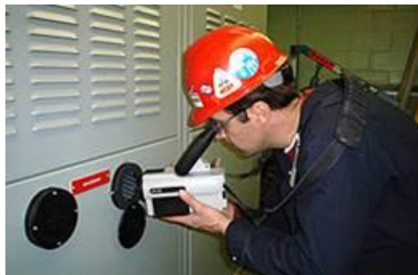
IR switchgear windows help to protect workers from electrical hazards.
