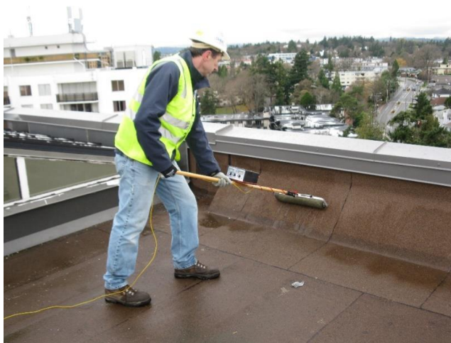
Figure 6: Low voltage vertical testing roller unit.
