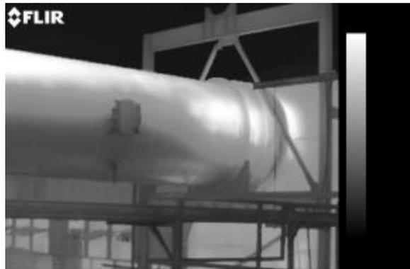
to adjust the thermal contrast by tightening the span. For restricted airflow in coal lines, a plug can overheat and spontaneously combust, causing an explosion.
