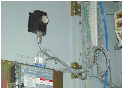
The ECM 586 ultrasound sensor mounted (left) and showing the output options (right)
