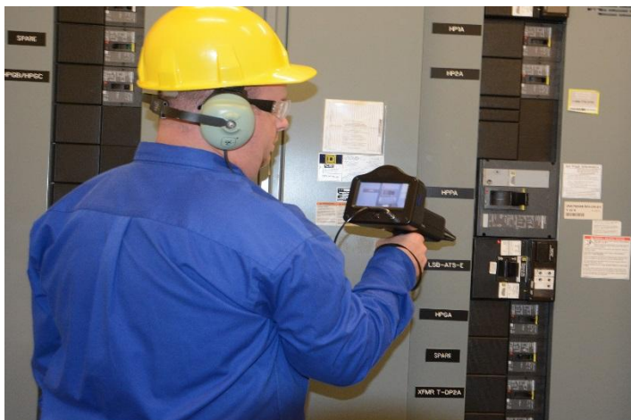
Traditional ultrasound inspection of enclosed energized electrical equipment
