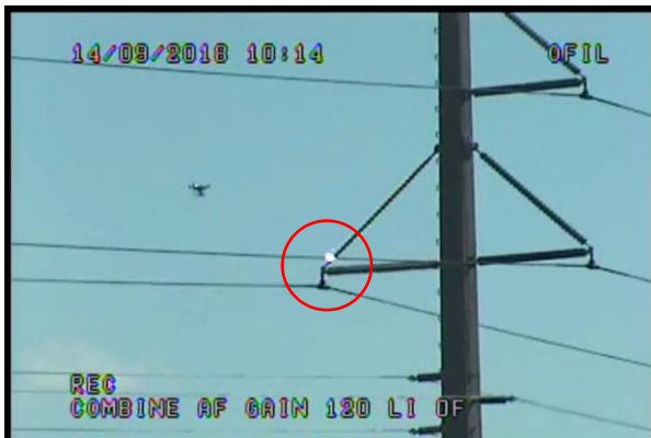
Figure 14: Left photo shows drone capturing visual images of where corona activity was detected on an insulator. Right image shows severity of damage with the fiberglass rod exposed and allowing water to infiltrate the interior of the insulator.
