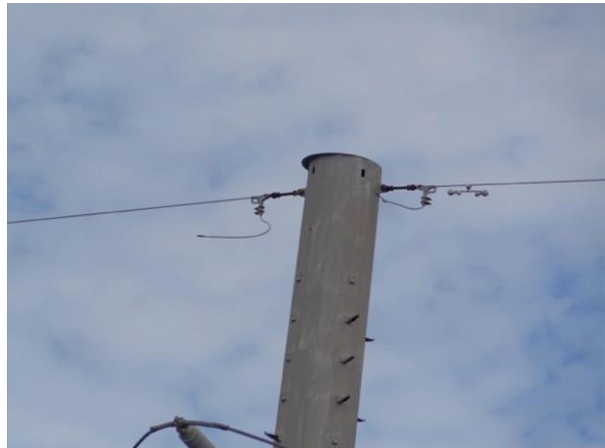
Figure 13: shows a hot spot detected on a static line connected via a dead-end to a metal pole. Note that the jumper wire is broken and causing the pole to be a new established grounding point.
