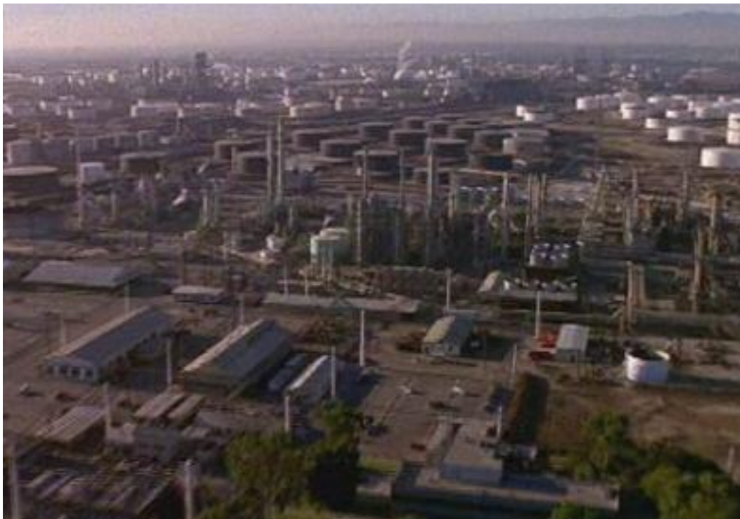
Figure 1. Petrochemical plants and tanks farms have thousands of potential leakage points
