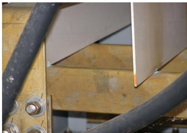
***Corona activity advancing to the tracking stage on insulation board resting on 13kV bus. Notice the carbon deposits and light brown discoloration of the insulation board on the right.***
